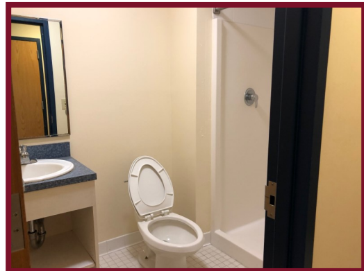
Bathroom - Vanity and Toilet
