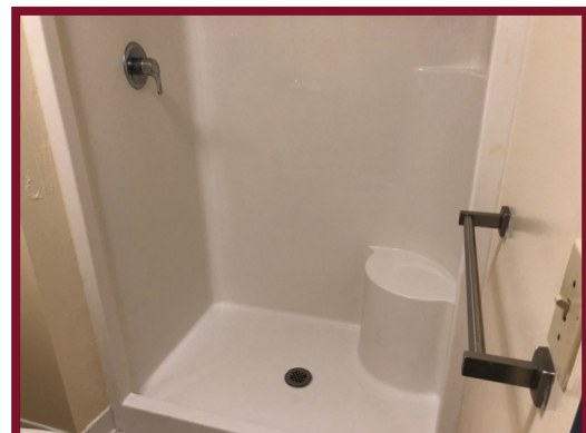
Bathroom - Shower Stall
