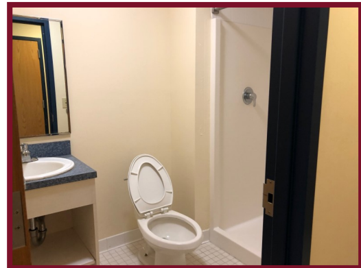
Bathroom - Vanity and Toilet
